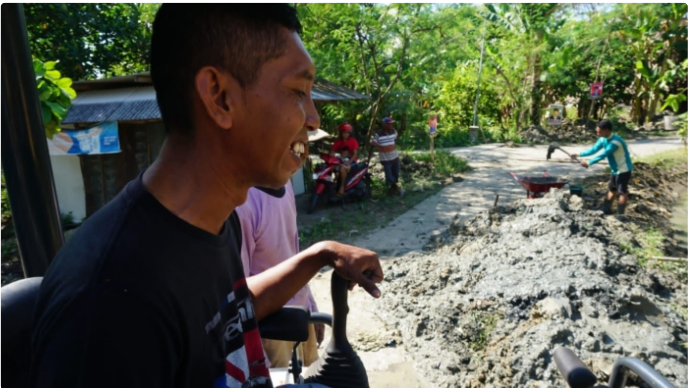
Sertu Abdul Aziz Sang Operator Excavator
